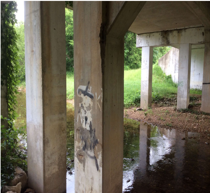
PHOTO 1 Description Bent #1 column #3 has 18" exposed rebar
