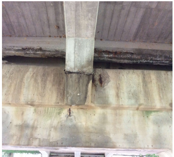
PHOTO 2 Description Bent #2 cap has 24" of rebar exposed
