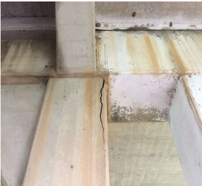
PHOTO 1 Description Bent #2 crack in column #4
