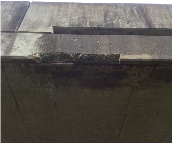
PHOTO 1 Description Right side span #3 soffit has 6' exposed rebar
