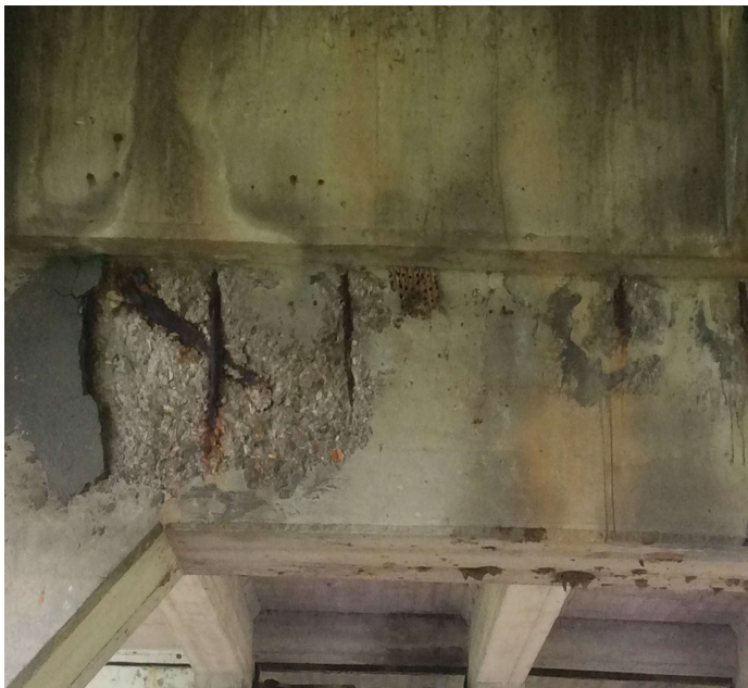
PHOTO 1 Description 5' exposed rebar to bent #1 cap
